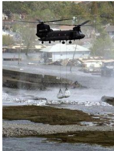
CH-47D drops sandbags to repair a breached levee in Louisiana on September 25 th , 2005
